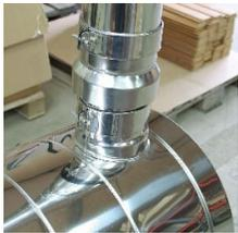
**Chimney Pipe holder** Fasten the chimney fitting. Then assemble the chimney pipe and put in place. NOTE! Turn the seam on the pipe backwards. **See pictures on last page.**
